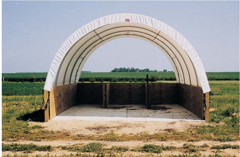
Hoop structure for composting with three bins.
