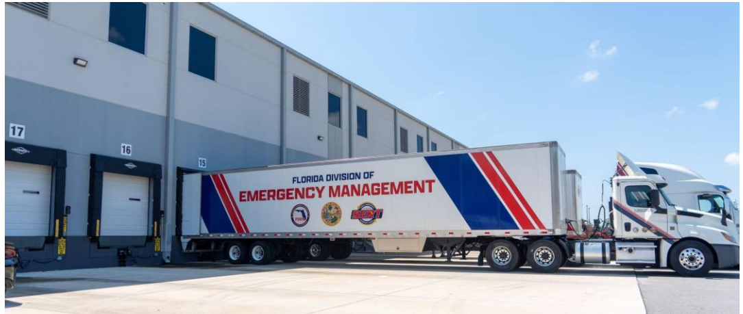
Florida Central Operations and Coordination Office (COCO) in Auburndale, Florida.
