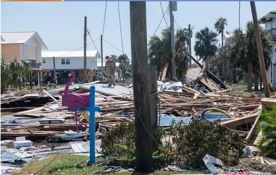
Damage in Keaton Beach, Florida, following Hurricane Helene. (Florida National Guard)
