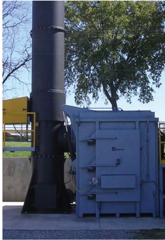
Figure 2–6. Fixed-facility incinerator. (Photo courtesy of FC Industries, Inc. Kansas City, MO)
