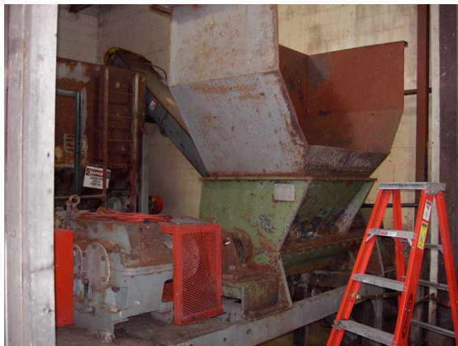
Figure 2-4. Both photos above show equipment in a rendering facility. (Source: Anderson, D.P., n.d)
